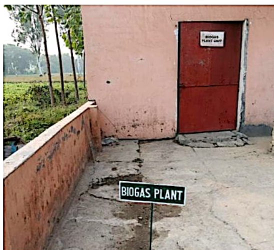
(Biogas plant in the university campus)
