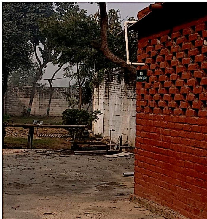
(Borewell and water supply network in the campus)
