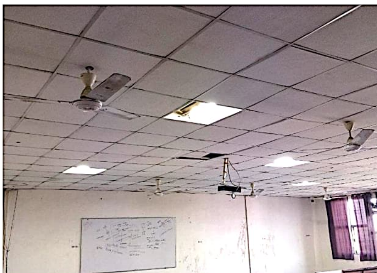
(LED lighting in the classroom of the university)
